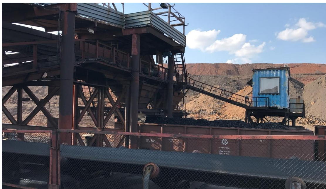
Figure 6-1: Centralny Screening and Coal Load-Out Plant – loading of screened Centralny coal to rail trucks
