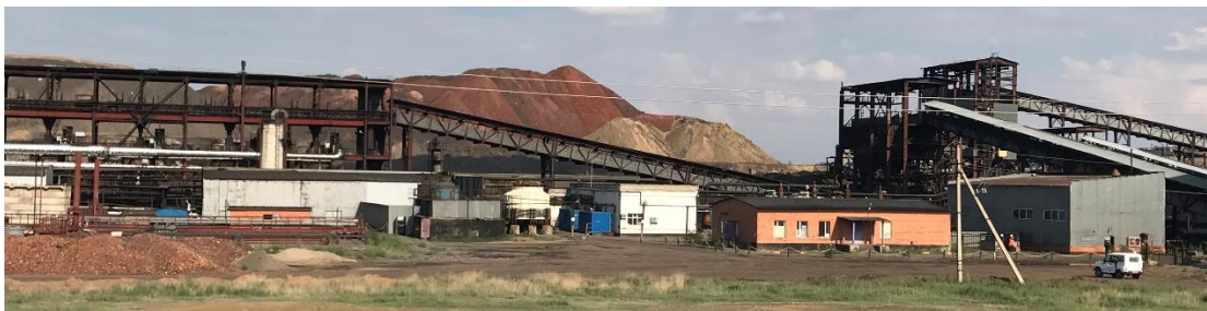
Figure 6-3: Sary-Arka Special Coke Plant
