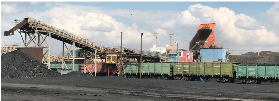
Figure 6-2: Zapadny Screening and Coal Load-Out Plant – direct loading of Zapadny coal to rail trucks via Conveyor No.1
