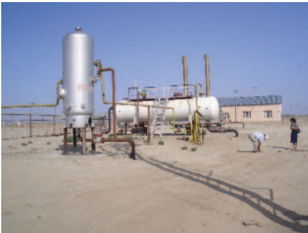
ZhaikMunaiGas NGDU Zhantalap Field First Stage Separator and Gas FWKO
