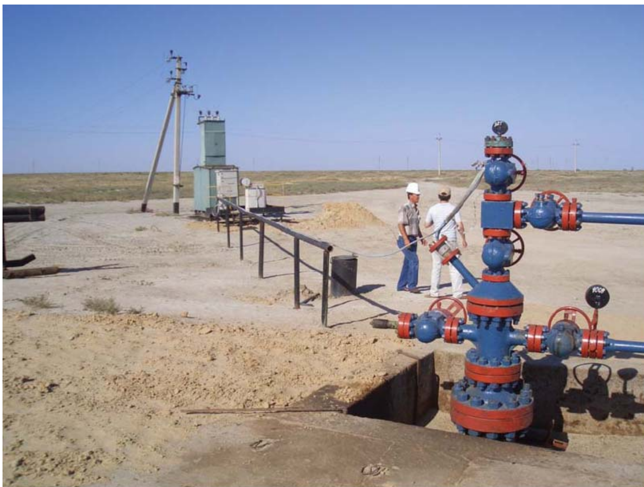
ProrvaMunayGaz NDGU Nurzhanov Field ESP Oil Well and Power Supply
